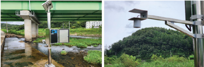
Flood prone road (Sejong City)
